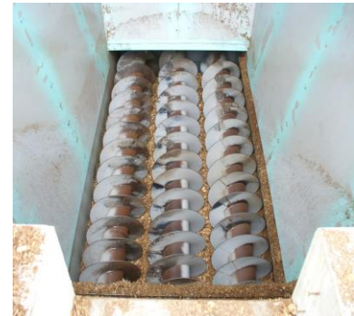
Mounting in discharge screw (wood-fired power plant)
